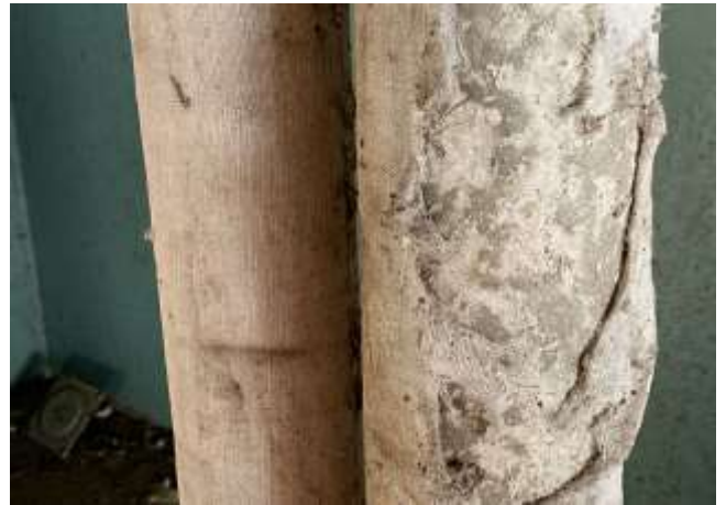
Thermal insulation of pipes with asbestos cloth
