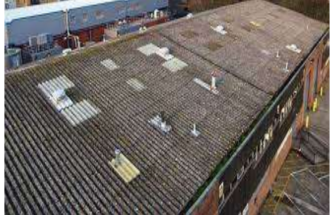
Asbestos roofing
