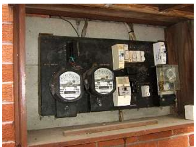
Asbestos in electric boards
