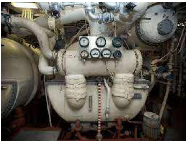
Generators with asbestos
