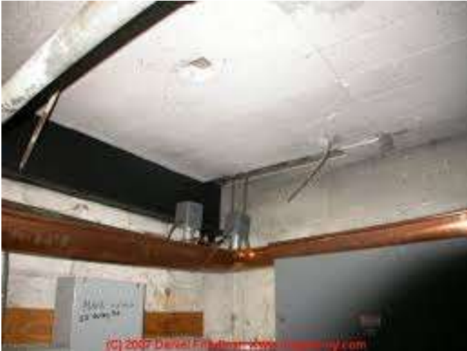
Asbestos plaster
