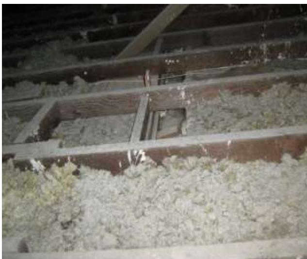
Bulk asbestos insulation made from unprocessed asbestos
