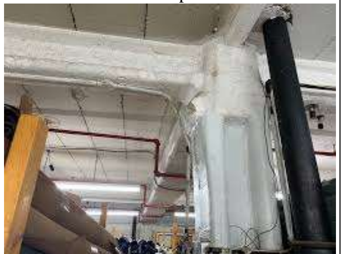
Asbestos panels
