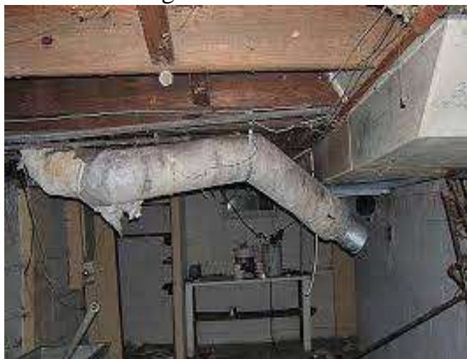
Heating ducts with asbestos
