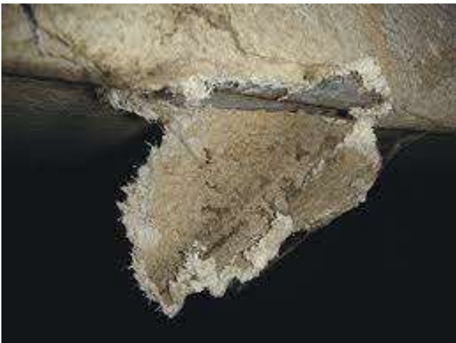
Asbestos duct insulation
