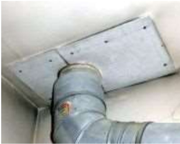
Panels from asbestos-cement tiles
