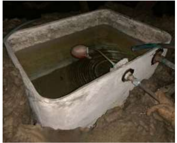
Water tanks made of asbestos cement
