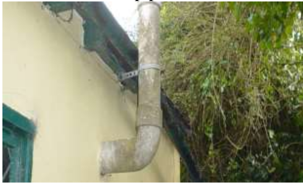
Chimneys from asbestos-cement pipes
