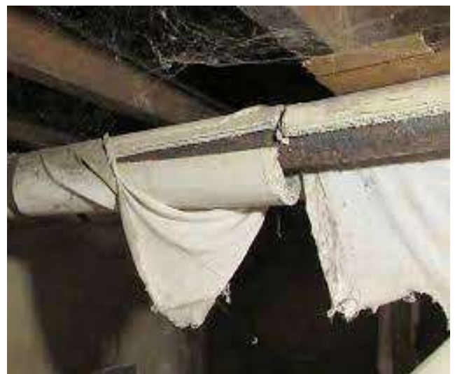
Pipe insulation or pipe lagging with ACMs
