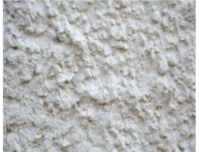
Asbestos popcorn ceiling covering
